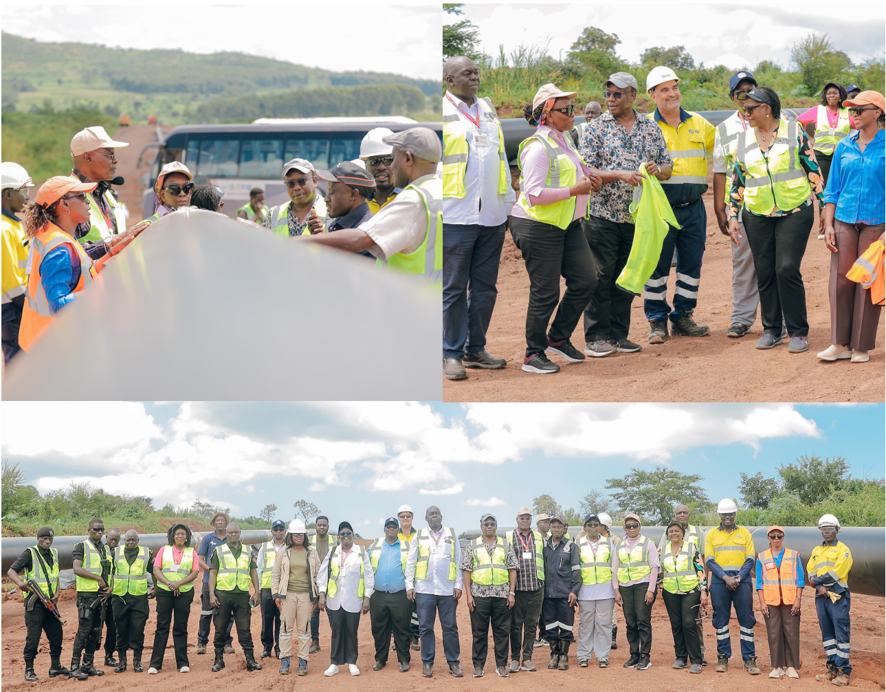
Members of the 6th Commission at the East African Crude Oil Pipeline site in Hoima City, November,2024.
